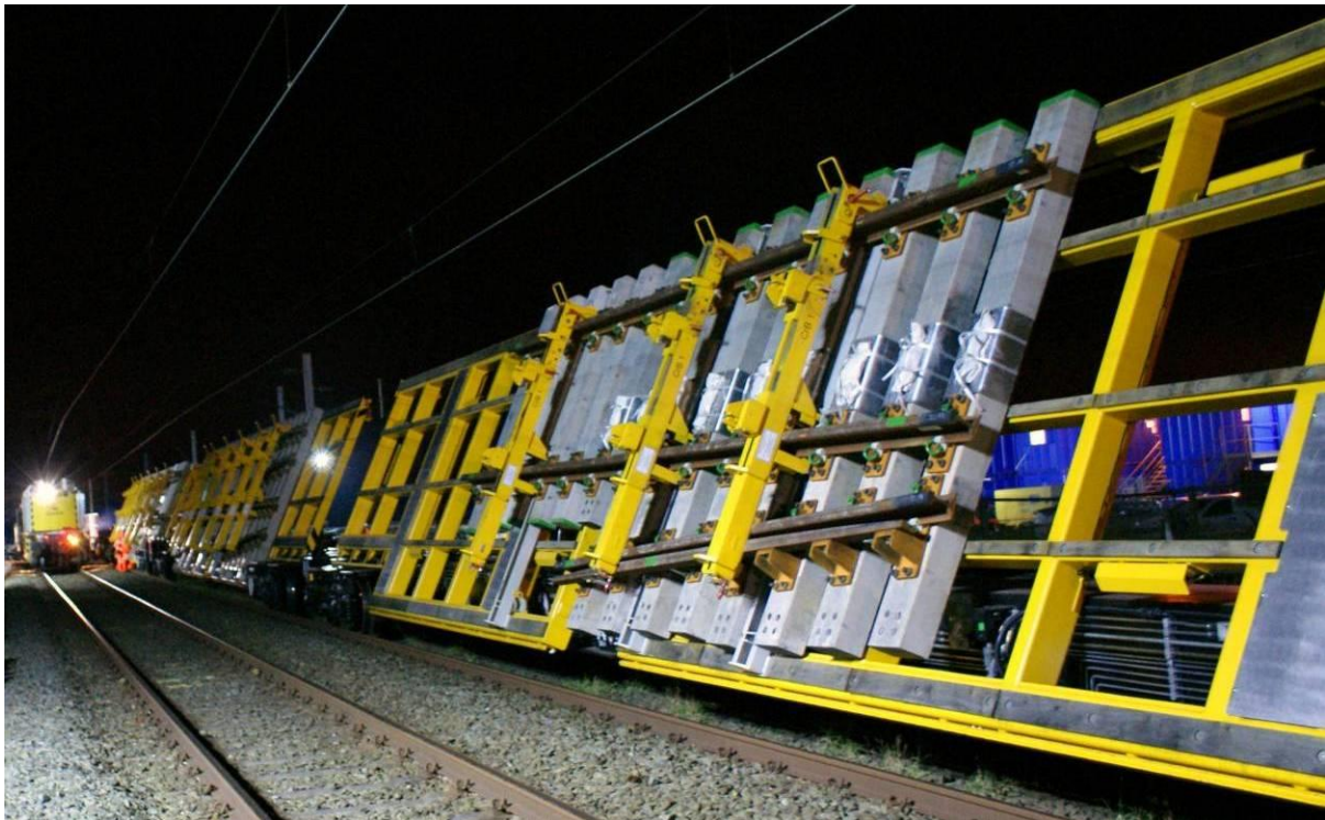
Figure 4. S&C panels ready to be lowered.
