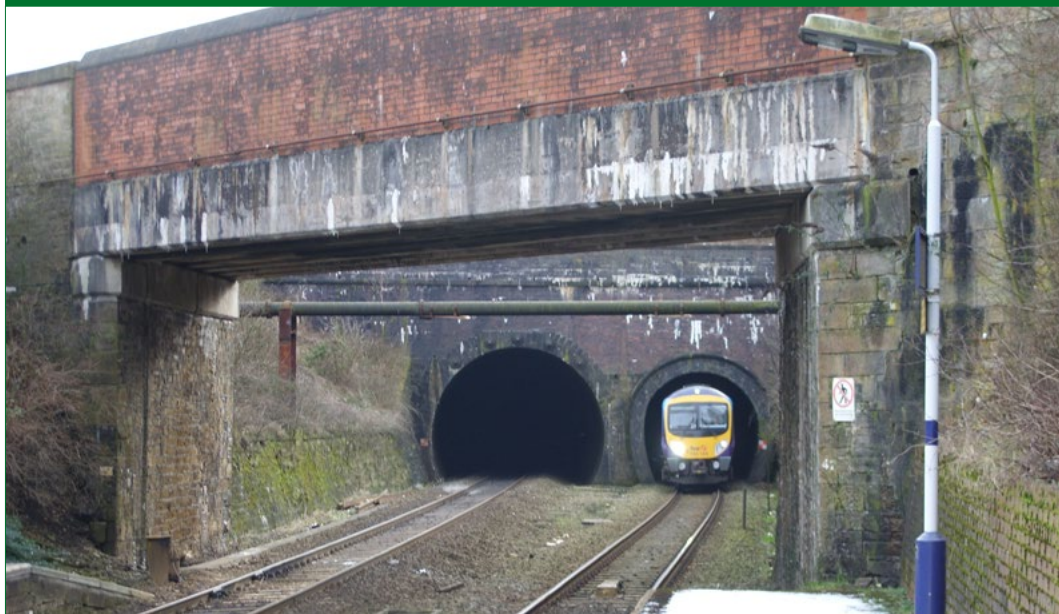
Figure 4.13 – Farnworth Tunnels part of the North West electrification project between Farnworth and Kearsley
