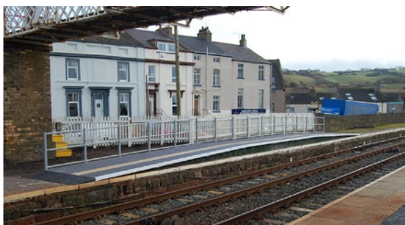
Figure E.1 Harrington Hump at Harrington station
