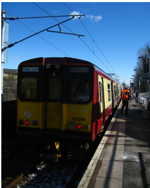
Figure 8.3 Paisley Canal station following completion of electrification
