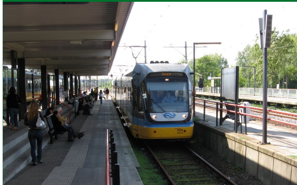
Figure 4.8 – Photograph of a low platform extension to accommodate a low floor tram train
