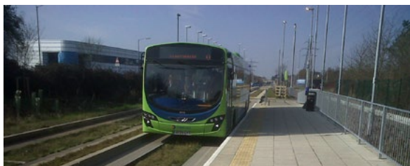
Figure 8.2 Cambridge Guided Busway
