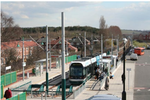
Figure 4.1 Photograph of Nottingham Express Transit Hucknall tram and heavy rail station
