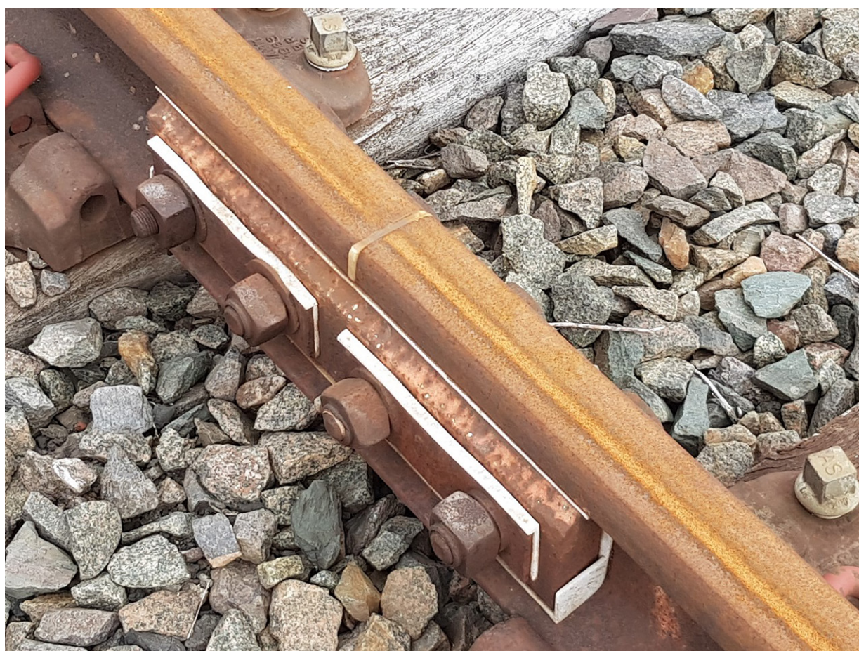
Figure 6: Insulated rail joint
