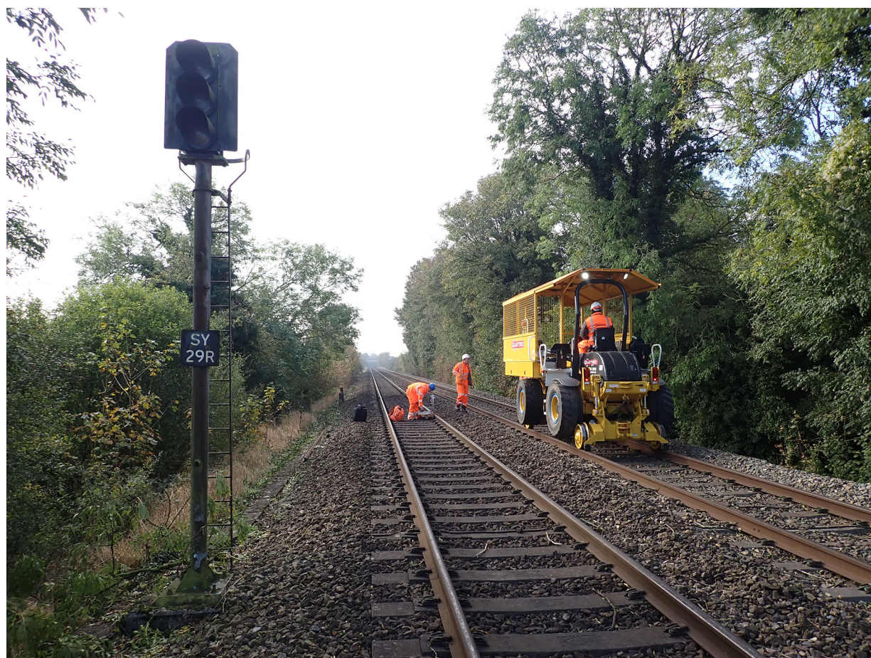
Figure 7: The railway at signal SY29R, looking towards Salisbury
