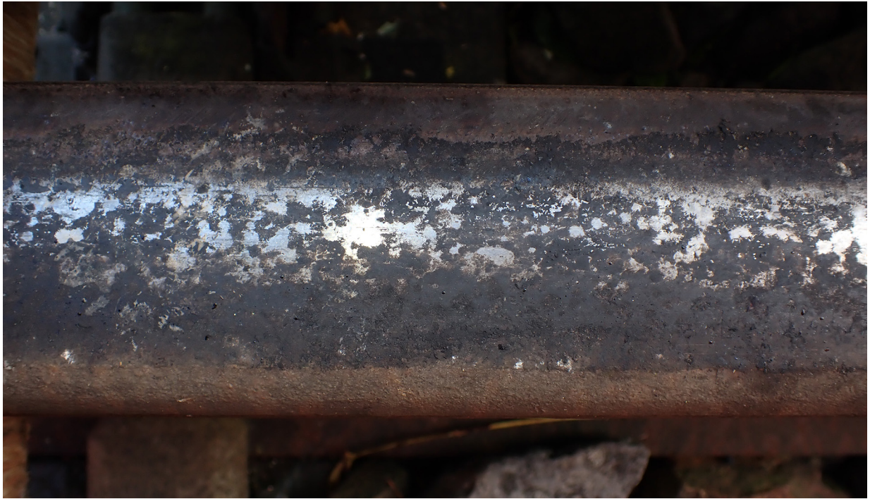
Figure 8: Railhead contamination on the down main line near signal SY29R
