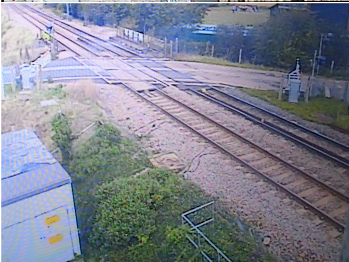
Figure 7: Photograph of the signaller's CCTV monitors for Enfield Lock level crossing (Liverpool Street SCC; top) and Ickleton Road crossing (Cambridge signal box; bottom)
