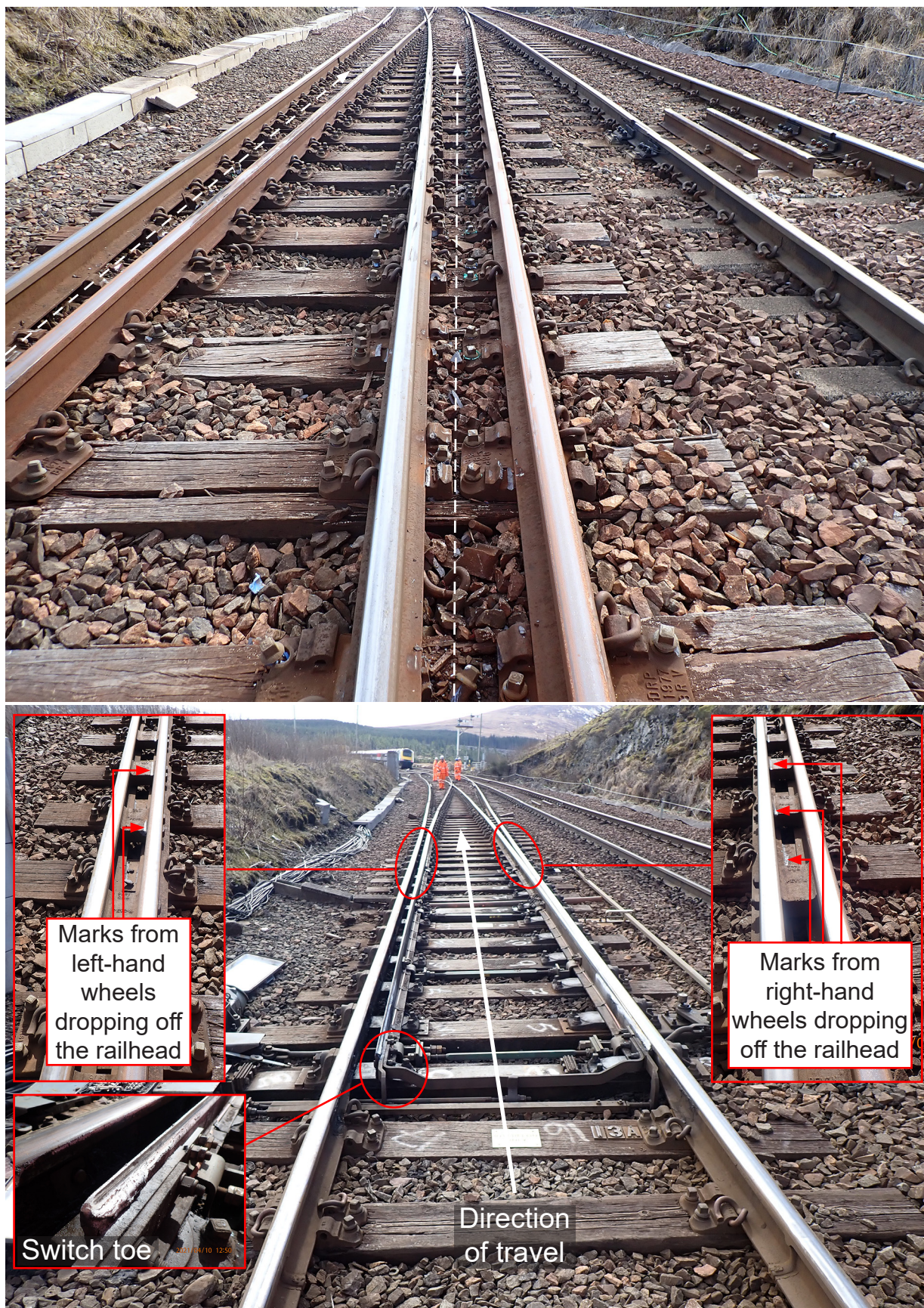
Figure 9: Derailment marks at 13A point end, switch rails in the normal position (as found after the derailment)
