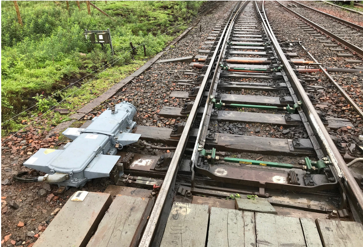
Figure 7: The newly-installed point machine at 13B point end (photograph courtesy of Network Rail)
