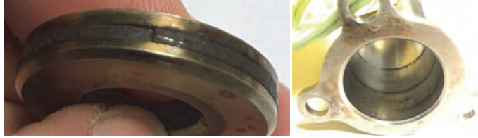
Corrosion found on piston and sleeve inner bore (Images used with permission of the operator)
