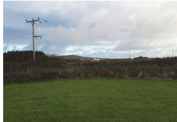
Power cables from approximately where the aircraft came to rest
