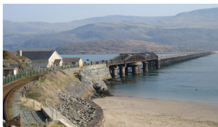
Barmouth Bridge (Photo: Network Rail)
