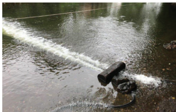
Bubble curtain in use (Photo: Network Rail).
