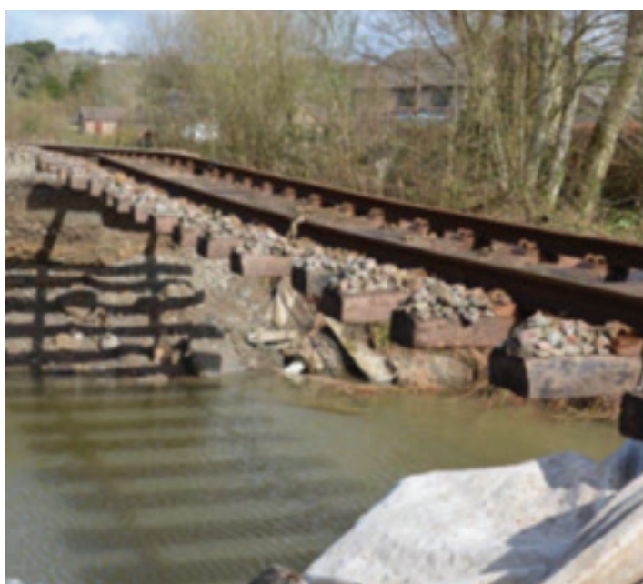
Image of the Conwy Valley line following the flooding incident in March 2019 (Photo: Network Rail)
