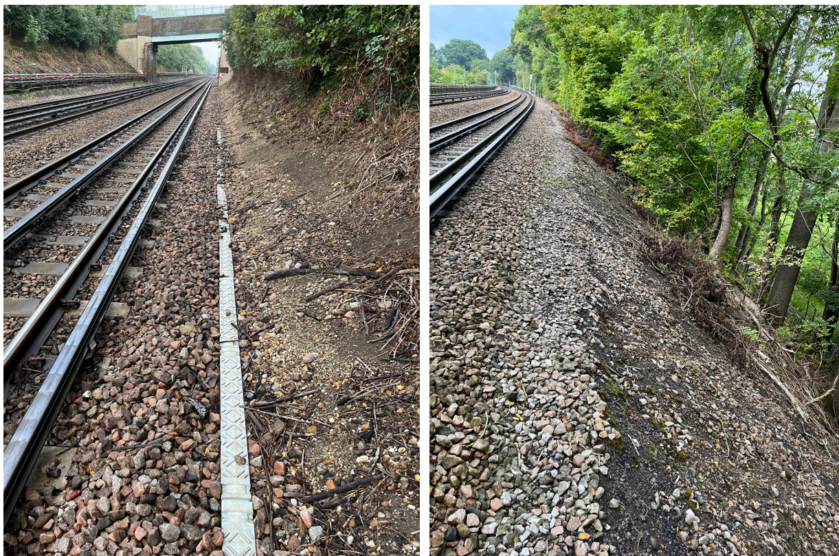
Figure 14: Photographs of the cess on the Metropolitan line north of Rickmansworth.
