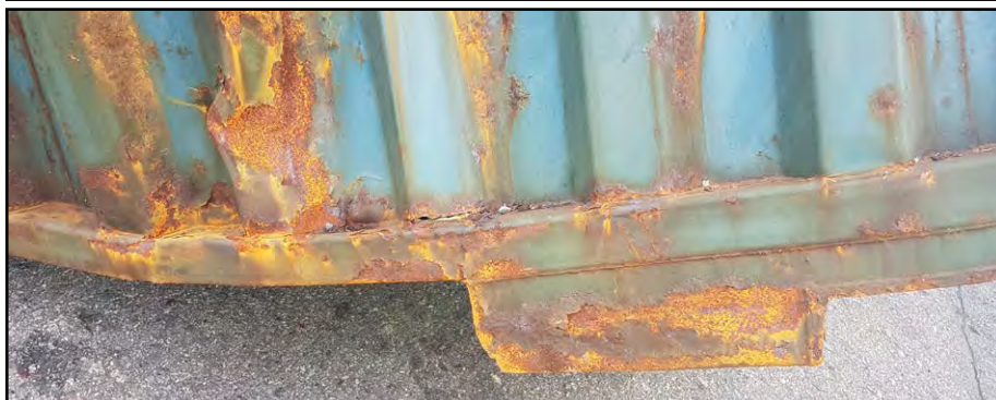
Figure 22: Visually apparent level of corrosion to the container stowed at the bottom of Bay 70's starboard outer stack
