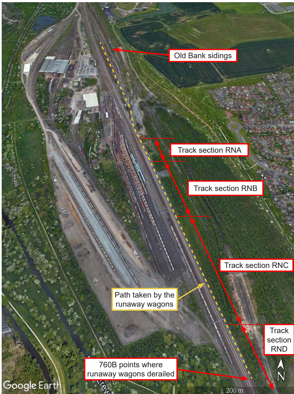
Figure 8: Track sections on the up and down independent line
