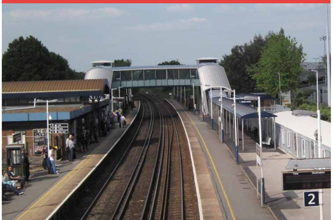
Photograph 20 – Southampton Airport Parkway new footbridge (taken from old footbridge)
