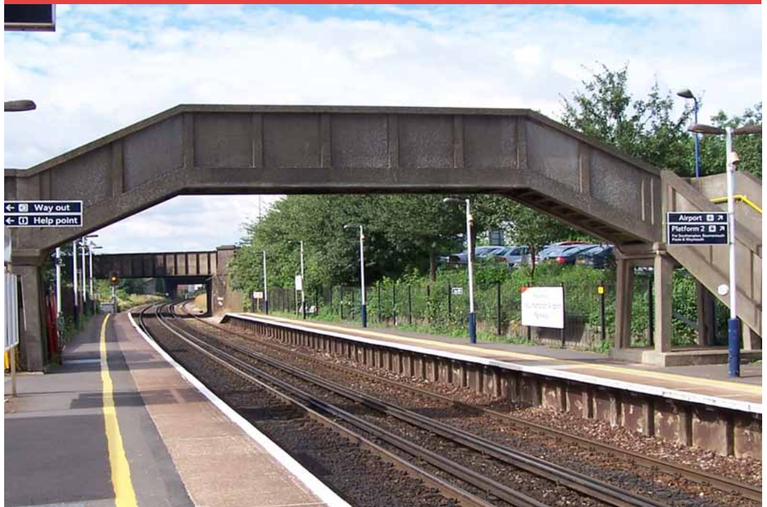
Photograph 19 – Southampton Airport Parkway old footbridge
