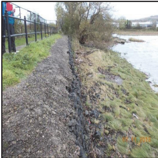
Photograph 2. Erskine North: Shoreline immediately to the east of Dumbarton Castle, with hard engineered pathway and eroding saltmarsh present
