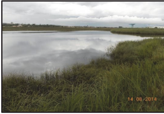
Photograph 10. Newshot Island: Tidal inlet at the downstream end of Newshot Island, with large expanse of existing saltmarsh habitat.
