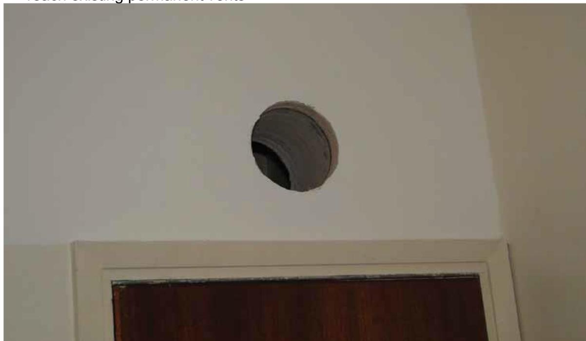
Figure 10 breach of fire-resisting enclosure
