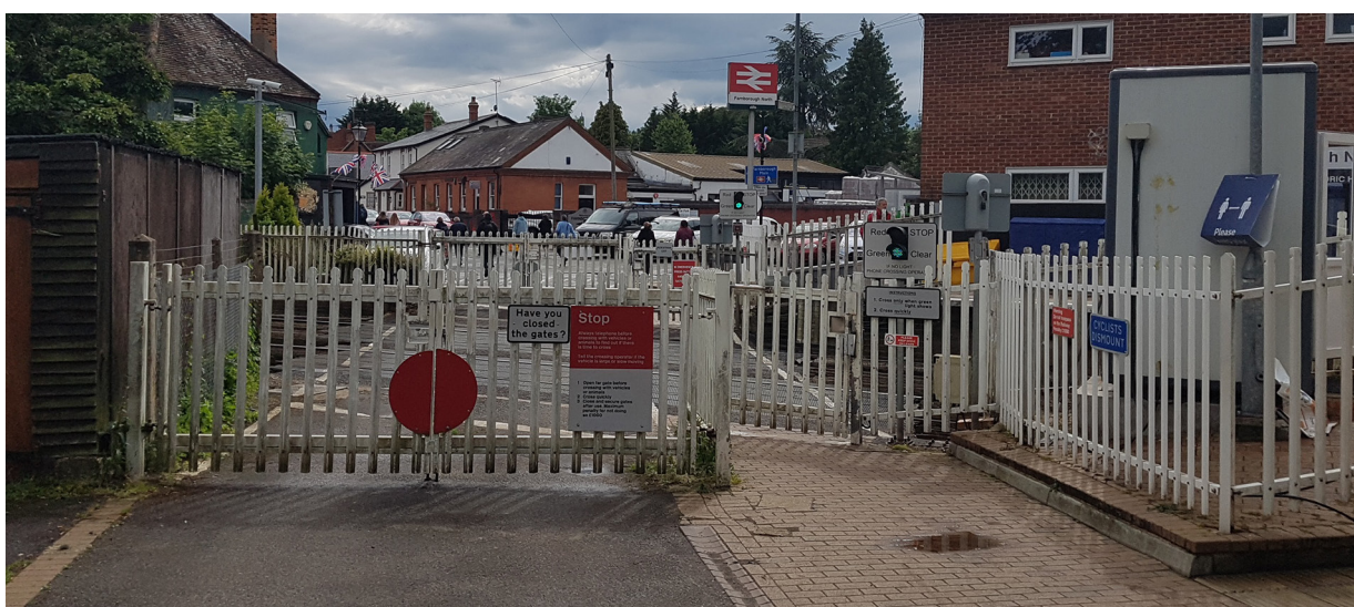
Figure 4: View looking west from near platform 1 showing user worked crossing (left), footpath crossing (centre) and side of crossing attendant's cabin (right).
