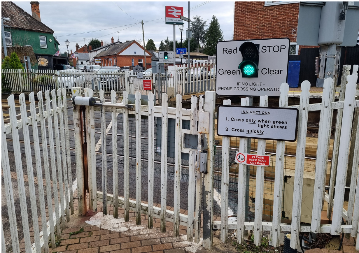
Figure 5: Footpath crossing gate near platform 1 with back-to-back miniature stop lights, visible on both sides of the railway.
