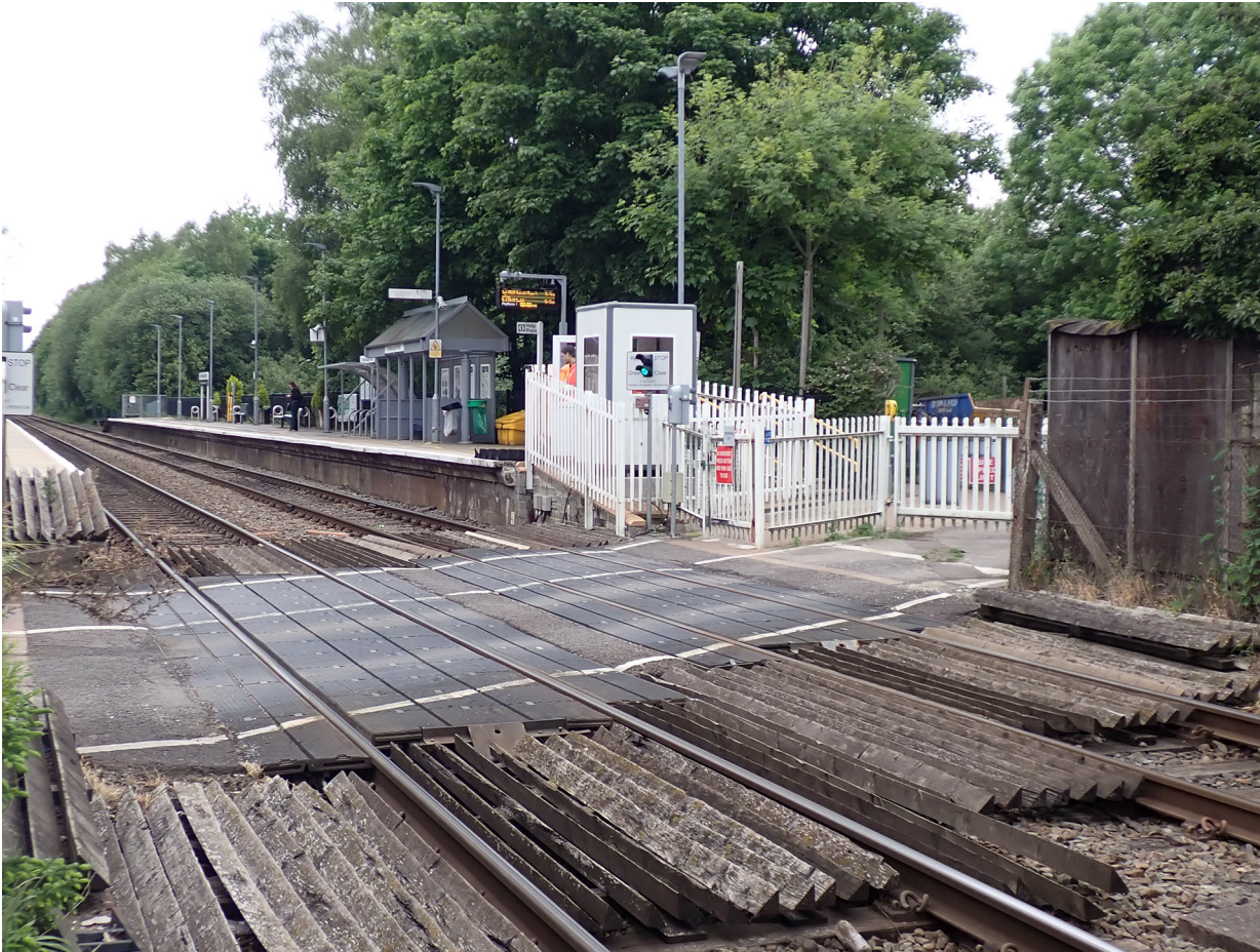
Figure 12: Crossing keeper's cabin within a fenced compound.
